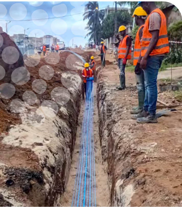
Laying pipes in Abidjan
